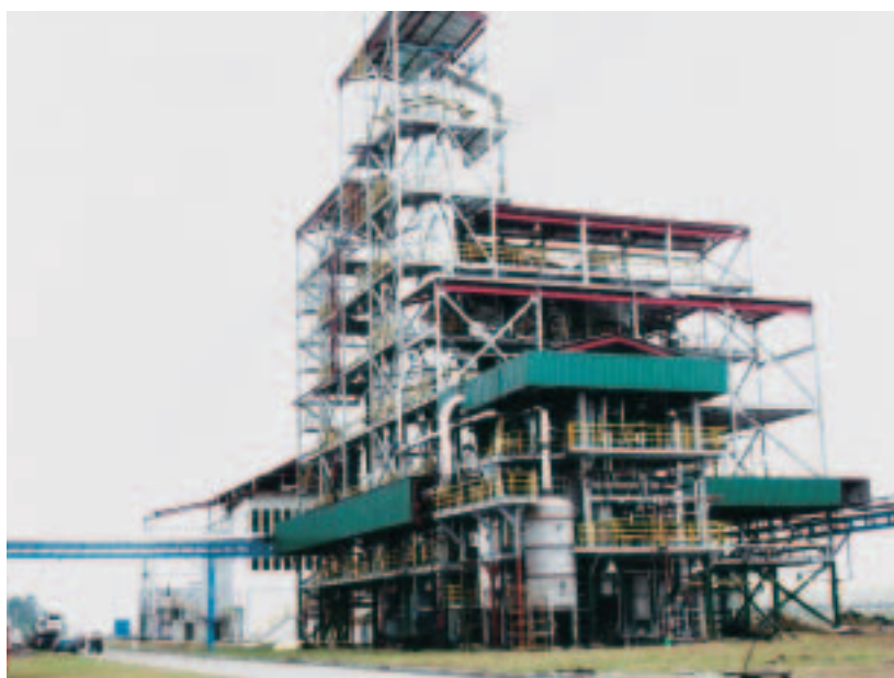
A state of the art fuel ethanol plant in Colombia, incorporating the latest in instrumentation and automation, executed with Exim Bank's support as a turnkey project by Praj Industries Ltd., a technocrat promoted company located in Pune. Attached to a sugar mill, the plant will process cane juice and molasses for production of ethanol.
